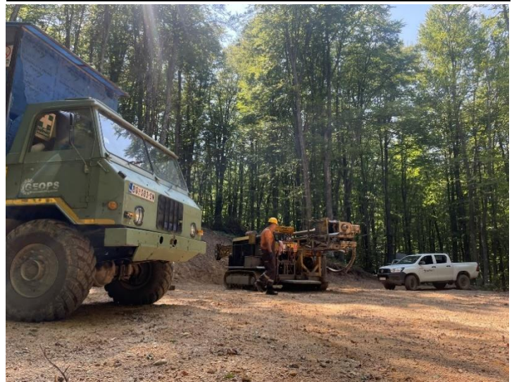
Figure 46: Site drill preparation at Shanac
