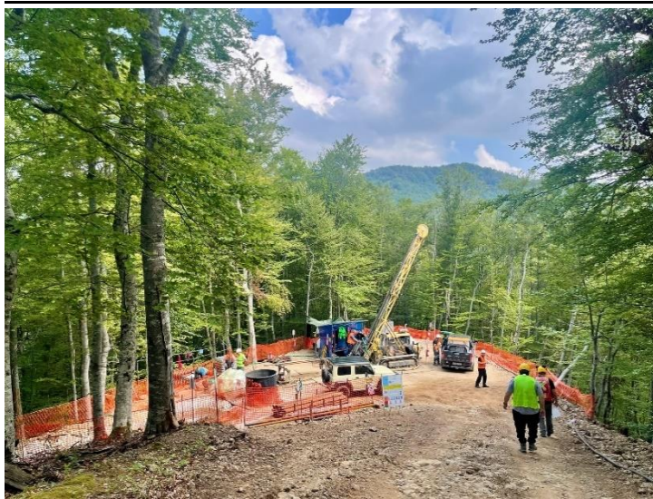
Figure 43: Drilling at Shanac
