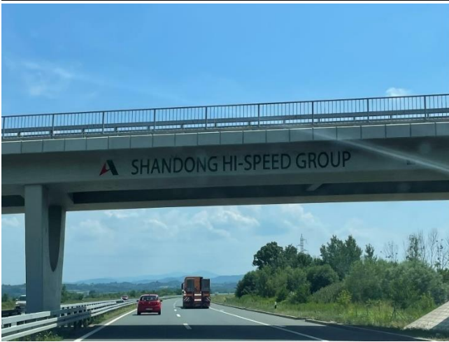
Figure 36: The highway constructed under the Chinese BRI
