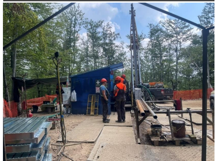
Figure 44: Drilling at Shanac
