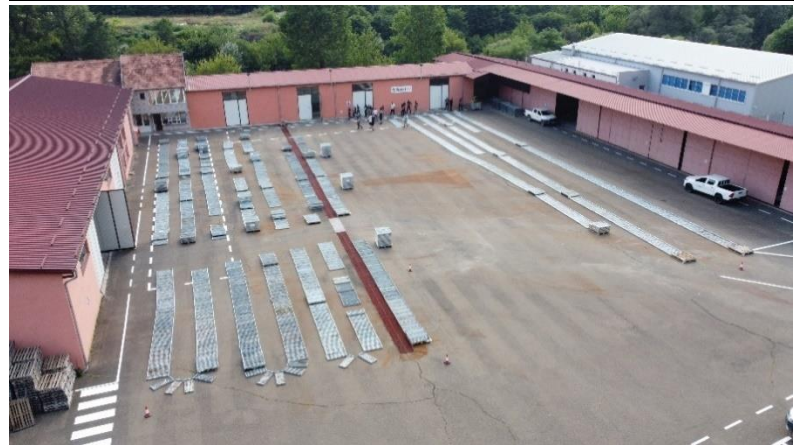
Figure 37: Overview of core yard facility in Raška
